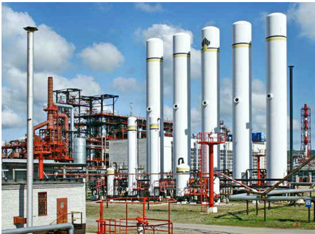
A major modernization project is going on at the Komsomolsk refinery
