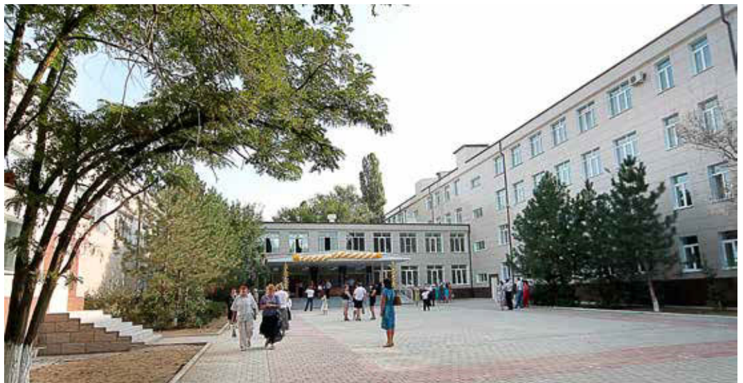
Neftekumsk school #3 after a major renovation
