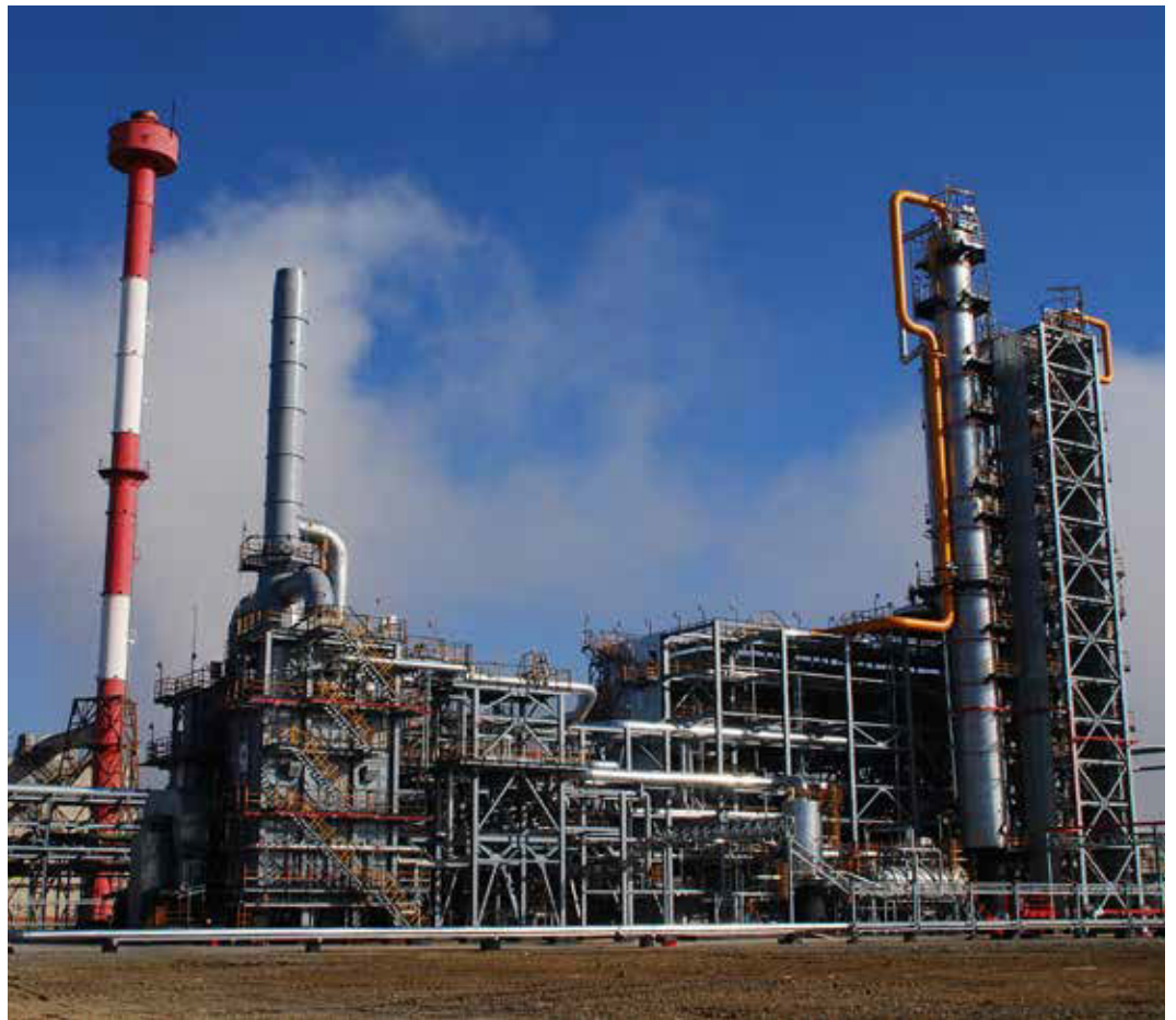
A gasoline prefractionation unit of the catalytic reforming plant at the Komsomolsk refinery
