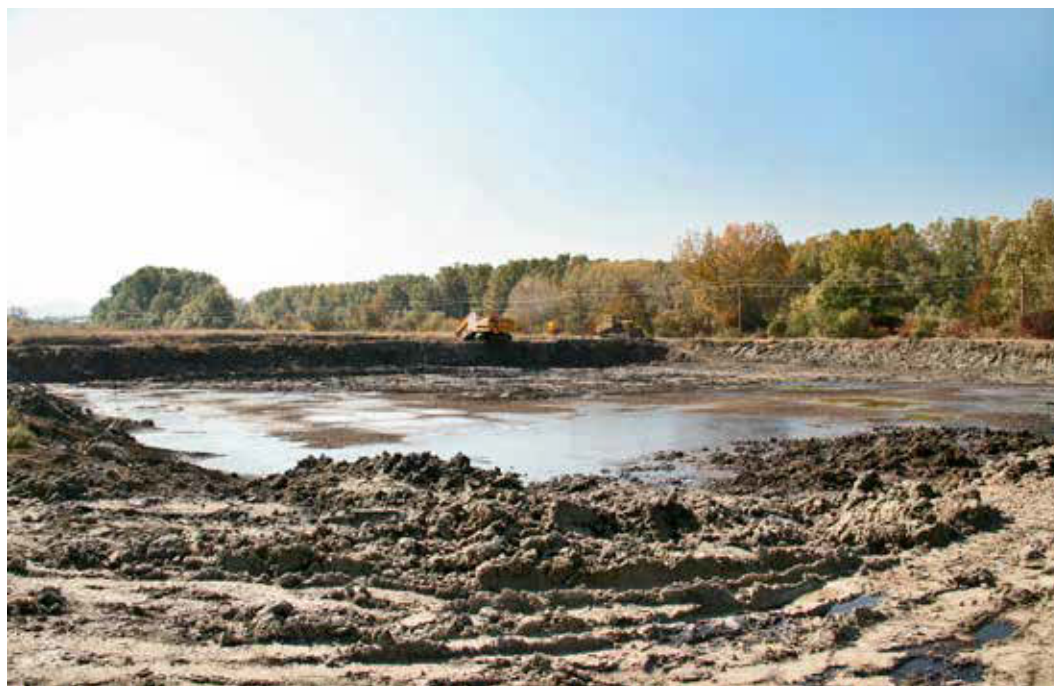
RN–Krasnodarneftegaz carried out works to prepare oil sludge pits and settling ponds for produced water for decontamination and subsequent reclamation
