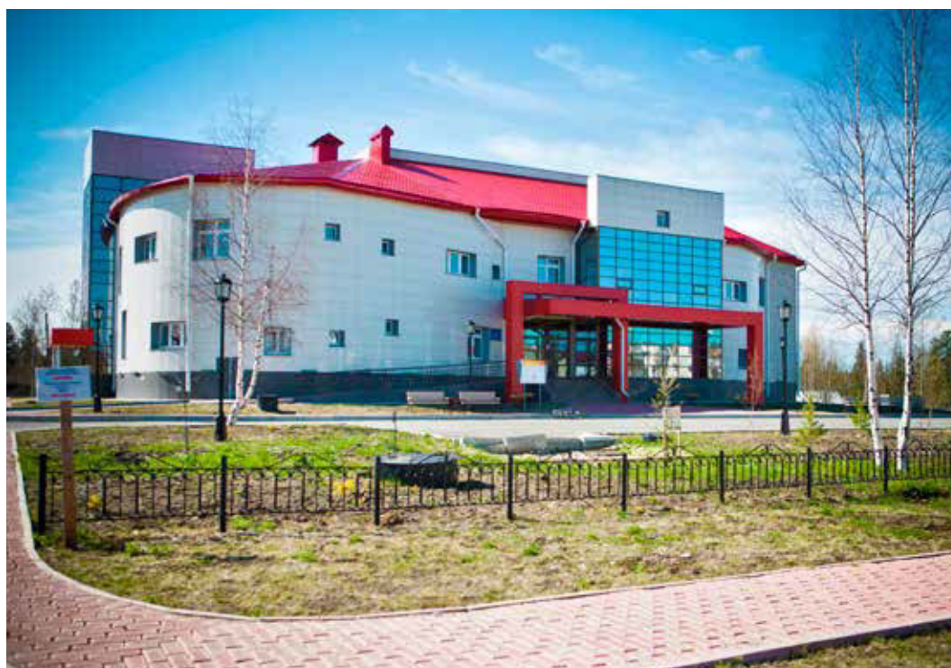
Construction of a new community center in Sentiabrsky (Nefteyugansk region, Khanty-Mansi Autonomous Area) was performed within the framework of socio-economic agreement between the Company and the District. The new community center, built using modern techniques and provided with all the necessary equipment, has become the hub of local cultural life
